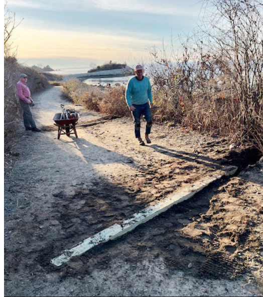
Bill Armstrong oversaw the planting of beach grass on the harbor-side bank (pictured, right) and the installation of water bars (left) to better divert water from the Knob access path.
